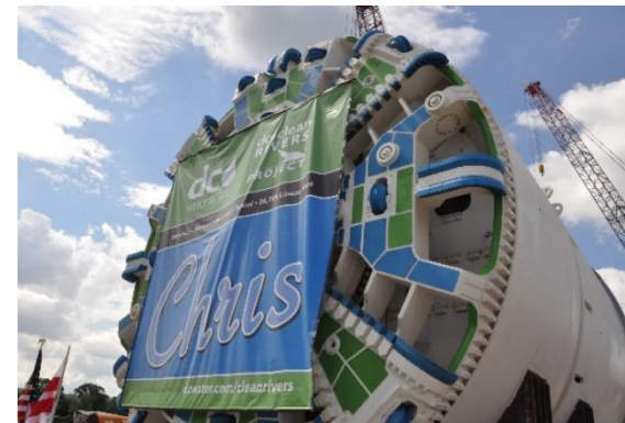
Anacostia River Tunnel
