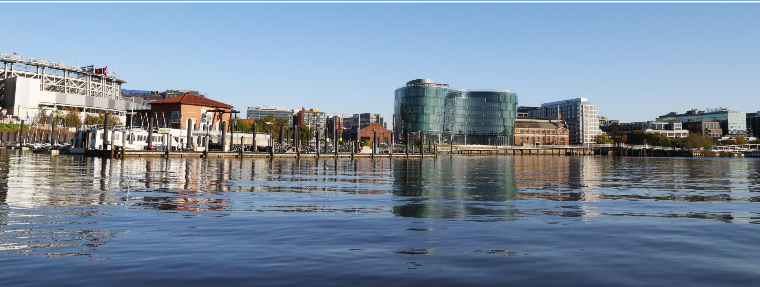
DC Water Headquarters from the Anacostia River
