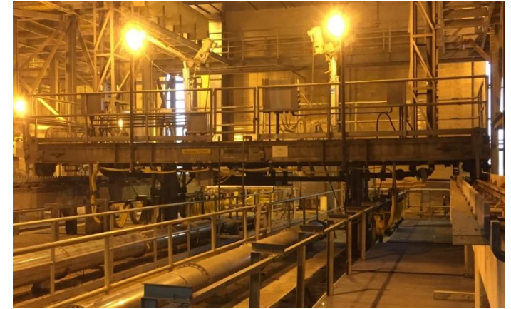
Screens, Grit & Primary Facilities Upgrades
